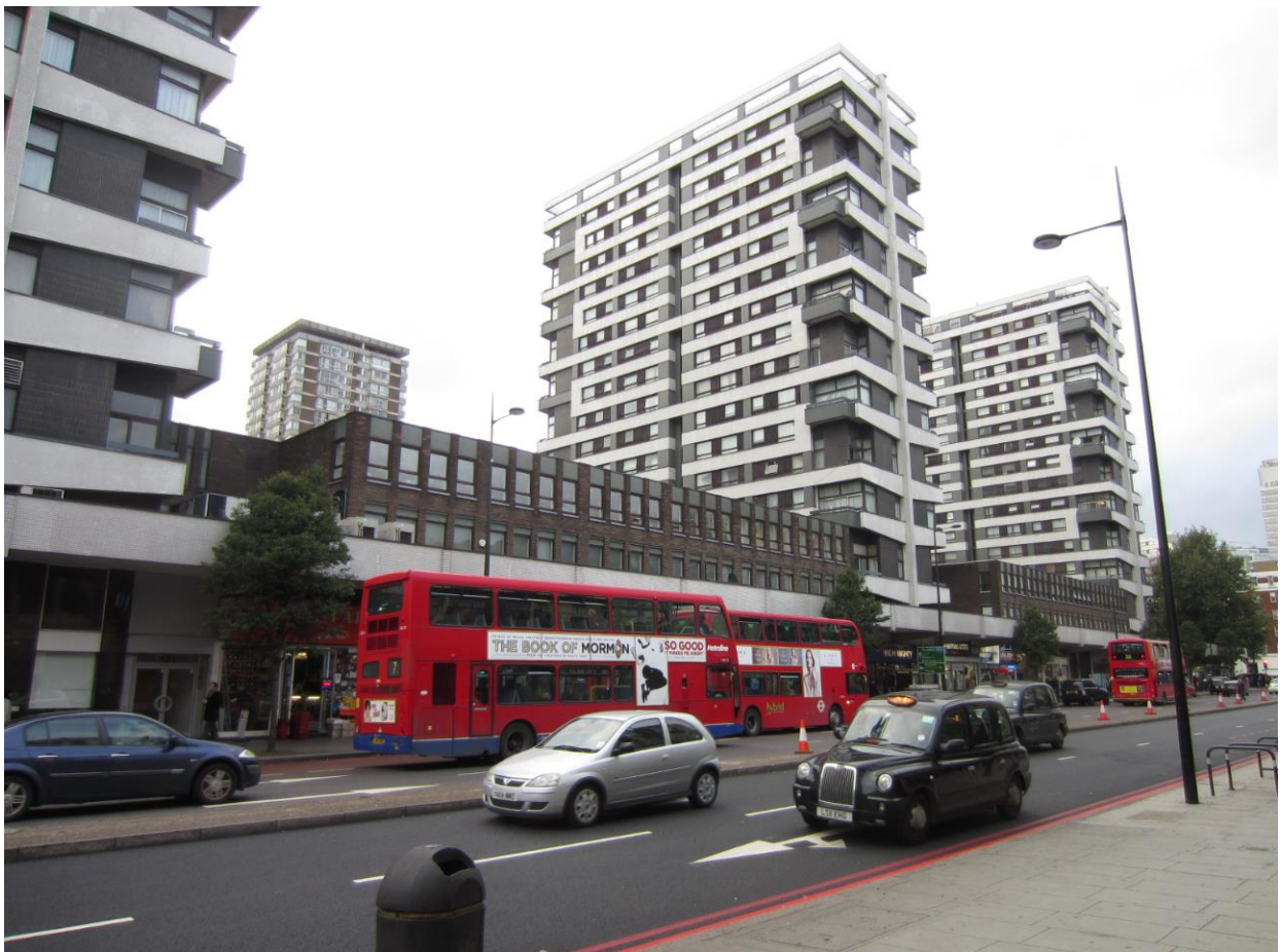
Front elevation from Edgware Road.
