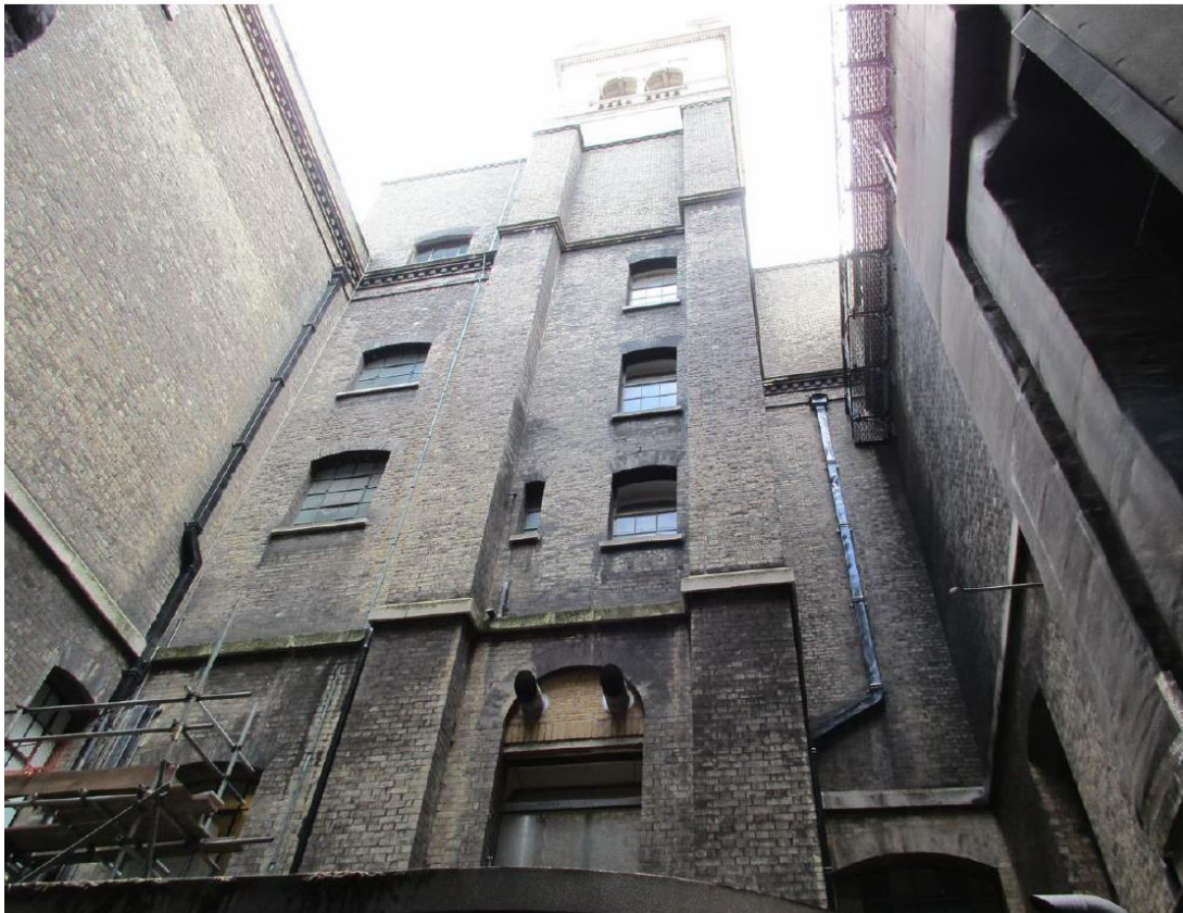
View of Belvedere Lightwell
